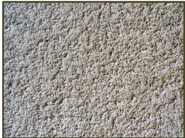
Example of a rough surfaced wall
